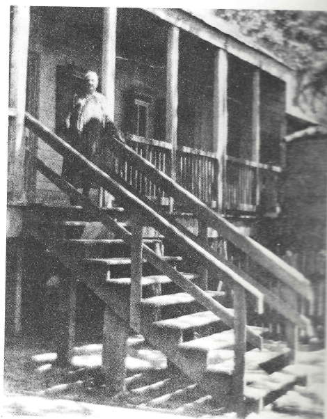
Larger houses, such as the Rigaud House pictured here, which was formerly on Grand Isle, were often raised because of the threat of floods. (From Jefferson Parish Yearly Review , 1943.)
