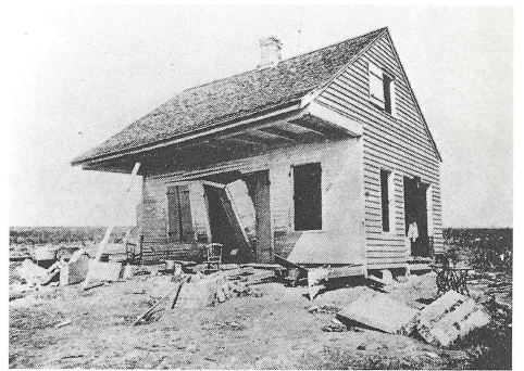
One of the best preserved houses left standing on Cheniere Caminada following the 1893 hurricane, a Creole type cottage. (From M. Forrest, Wasted by Wind and Water . Courtesy Special Collections Division, Tulane University Library.)
