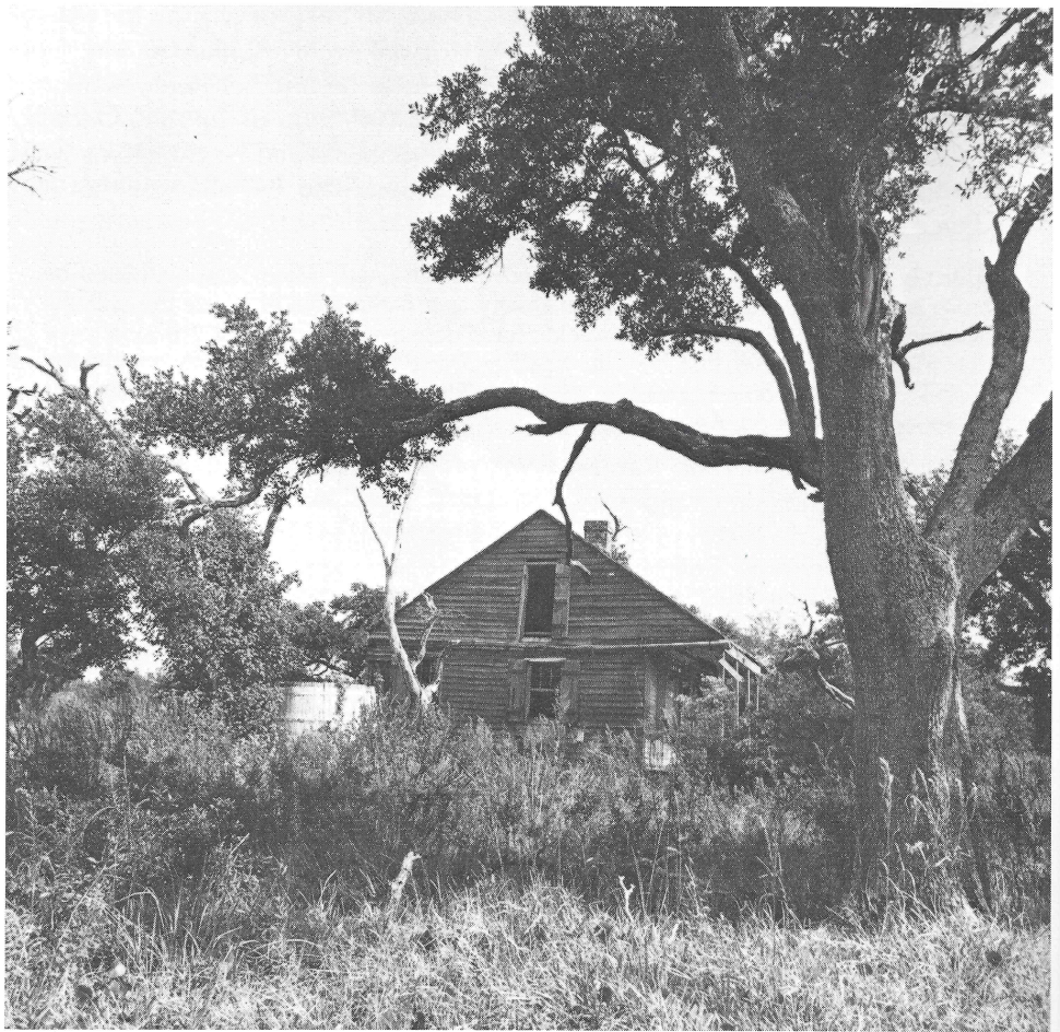
An abandoned Creole type cottage on Grand Isle, having a cypress shingle roof, batten shutters, and a cistern.
